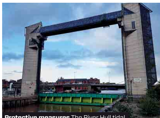
Protective measures The River Hull tidal surge barrier in Kingston-upon-Hull
